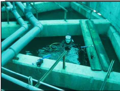
Kevin is performing an underwater structural inspection of the deteriorating fountain.
